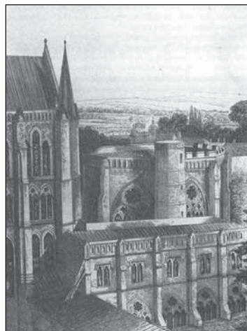
17th century view showing crenellations (Hall)
